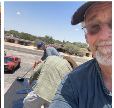
Sometimes our evangelists do more than teach – Jim helped with roof repairs at the Tanglewood church of Christ (Odessa, TX).
